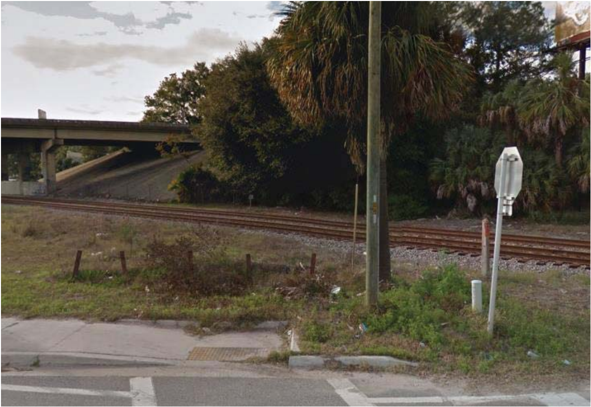
Railroad tracks and overpass across College Street and Willow Branch Avenue
