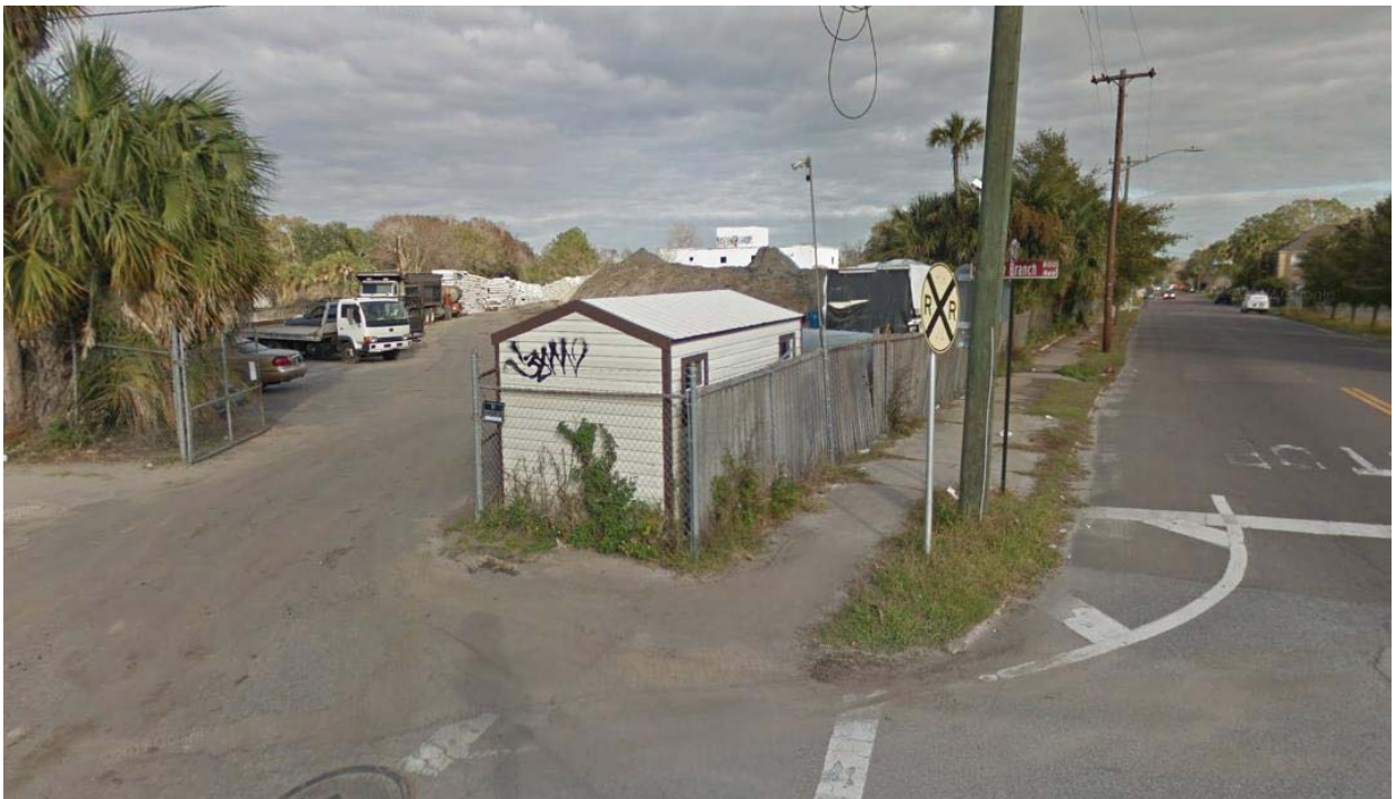
Industrial complex across College Street
